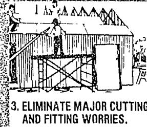
2. INSTALL THE PRE-BUILT ROOF TRUSSES
