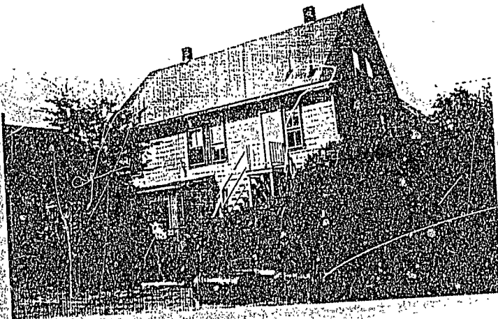
REAR VIEW OF REAR BUILDING
