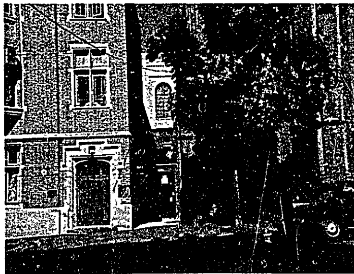
Pre-construction facade at alley
