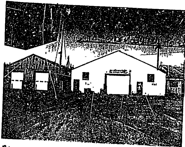
PHOTO TAKEN IN SOUTHWESTELY DIRECTION 135 MARGINAL WAY, PORTLAND, MAINE 6-14-94
