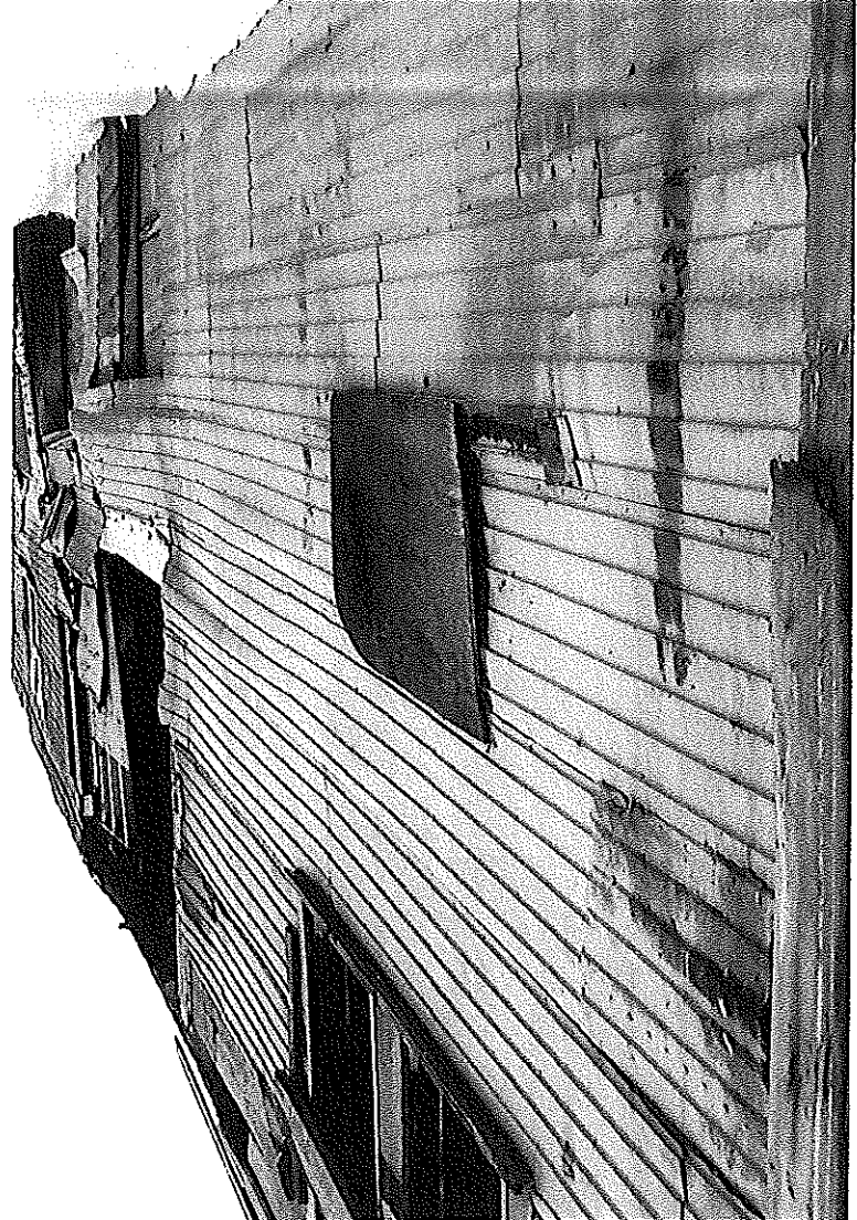
Back (Water) side
