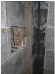
KISC has begun demoing the delaminated concrete at the lobby concrete slab at each level, see photo below. The exposed reinforcement has good concrete cover but shows signs of corrosion. KISC is to clean and coat the reinforcement and place the concrete repair material flush with the existing surfaces.
