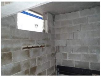
10. KISC is continuing to grout the vertical reinforcement within the stair and lobby interior. See adjacent photo.
