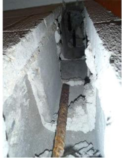
8. KISC has exposed varying cell conditions. Some of the cells are reinforced with and without grout or are partially grouted. At the majority of the reinforced locations adequate laps lengths were not provided during original construction and gaps between the rebar were observed. See photo above. KISC noted that at one location a bunch of 8 foot lengths of rebar were stuck into an ungrouted cell.
