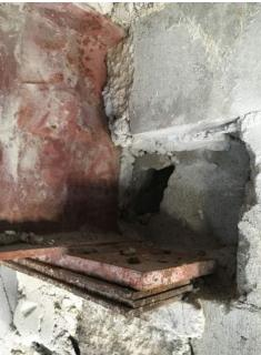
5. KISC has saw cut and removed material from approximately 80% of the vertical cells. See photo below. KISC has begun to install vertical reinforcement within the cells. Spot checks of the rebar laps lengths were performed. If the existing rebar is in good condition and is in the correct location within the cells it is to be reused. Forming and grouting of the vertical cells is anticipated to take place next week.
