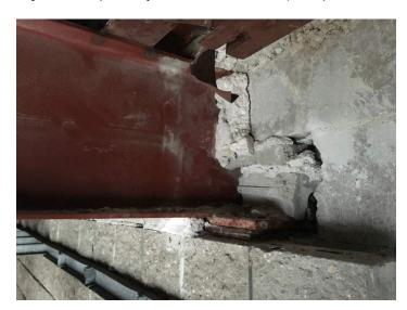
3. BSE's noted that the exposed steel angle door lintels at the grade level are in good condition and do not have to be replaced. All exposed steel should be cleaned, prepped and coated. The existing lintels have a large bearing length (8" to 12") and potentially interfere with the proposed vertical reinforcement. BSE to provide KISC with guidance. (See photo below).
