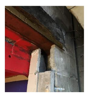
4. KISC removed the spilt face block façade at the high steel beam picking up the sloped roof members between the tower and ferry terminal. The beam was found to be bearing on the CMU wall approximately 4" +/- and partially on the split face facade. The lower steel beams extending from the HSS column and bearing into the CMU wall are in fair to good condition. Rusted sections need to be cleaned, prepped and coated. (See photo below).
