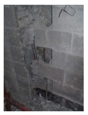
7. KISC has begun to open the face shells of the CMU block to install vertical reinforcement in the stair tower. Of the three areas opened two were fully grouted and one was partially grouted. None of the CMU cells had any vertical reinforcement within them. (See photo below).
