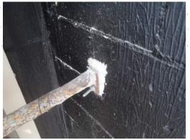
10. Before the wall panels are installed, the exterior needs to be washed down to remove debris so it isn't stuck behind the siding once installed. See photo below
