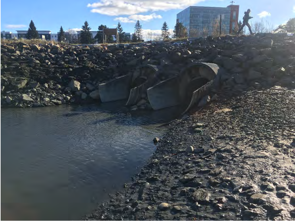
Photo 4 – Storm drain outfall into Back Cove.
