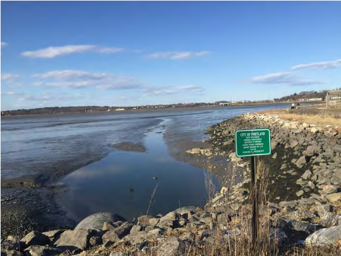
Existing twin 84" combined sewer overflow outfall facing north
