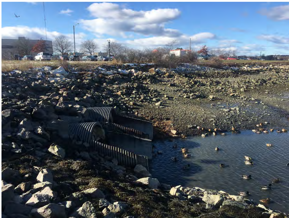
Photo 2 – Storm drain outfall into Back Cove, facing west.
