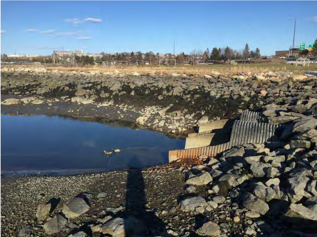
Existing twin 84” combined sewer overflow outfall facing east
