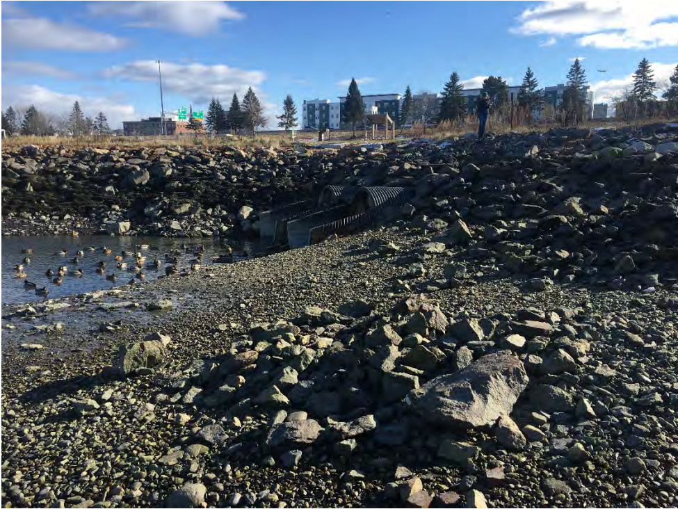
Photo 3 – Storm drain outfall into Back Cove, facing east.
