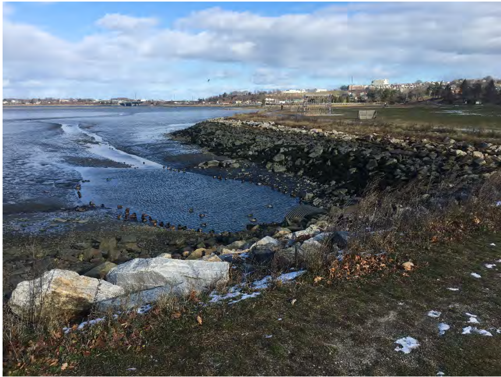
Photo 1 – Storm drain outfall into Back Cove, facing north.
