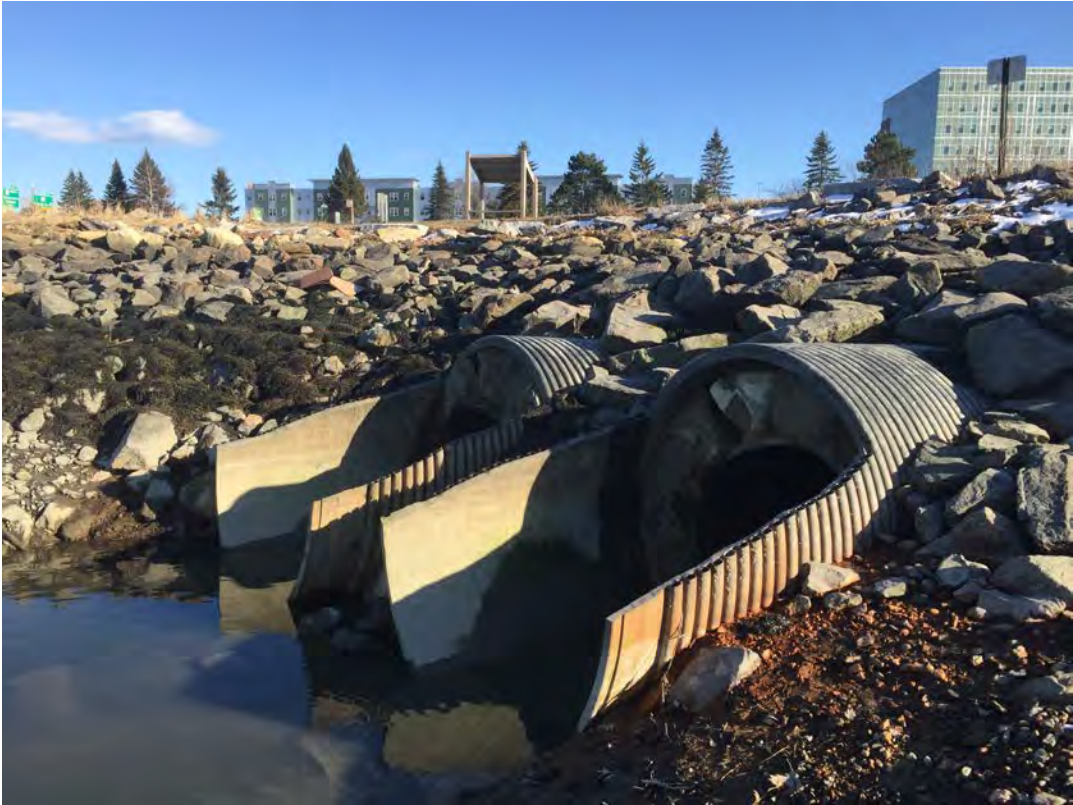
Existing twin 84” combined sewer overflow outfall facing southeast
