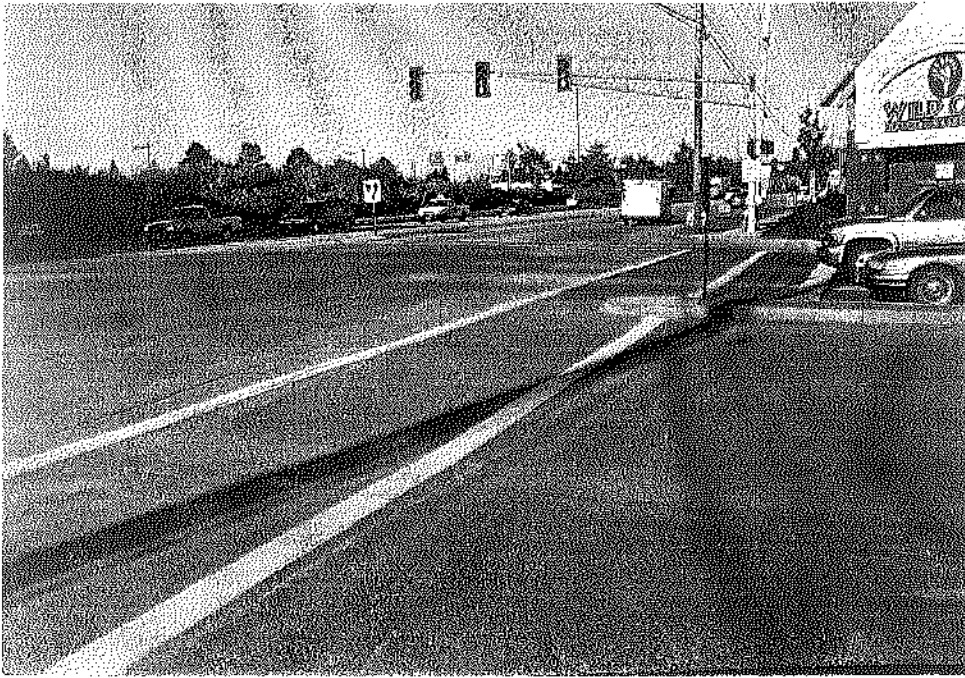
MARGINAL WAY LOOKING NORTHEAST FROM BANK
