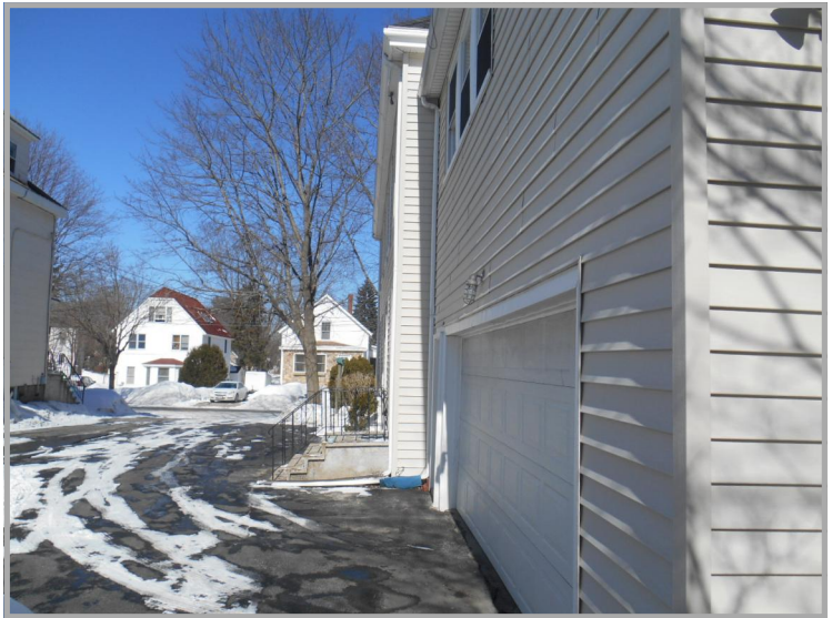
Additional East Side/Rear View
