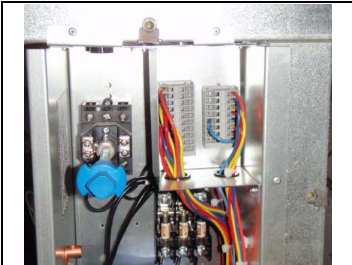
FIGURE 4-5 TERMINAL BLOCKS FOR CONTROL DEVICE CONNECTION.
