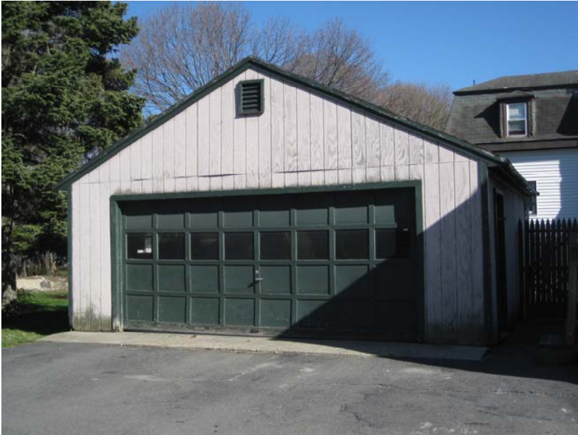
51 Olympia St – Garage to be Demolished (North)
