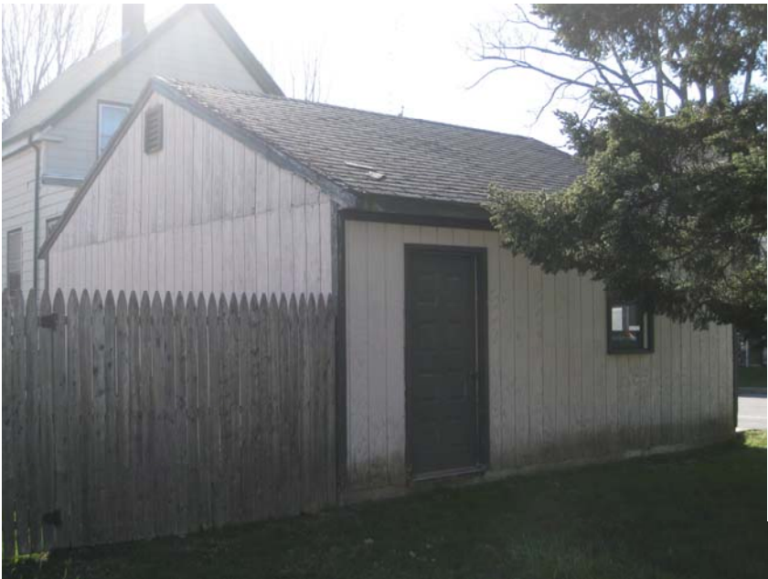
51 Olympia St – Garage to be Demolished (East)
