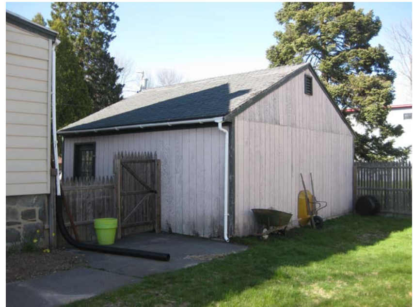
51 Olympia St – Garage to be Demolished (West)
