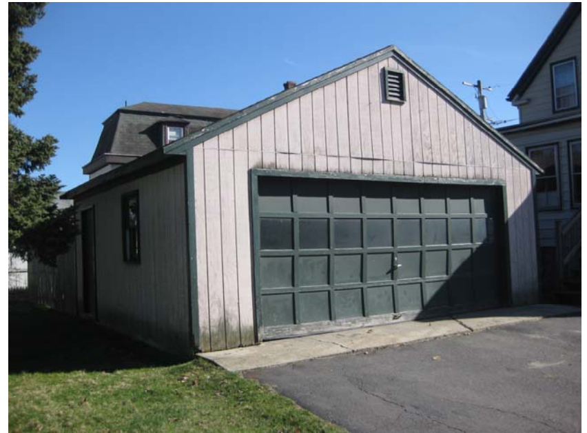
51 Olympia St – Garage to be Demolished (North)
