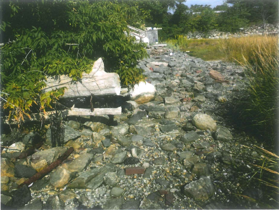
Photograph #3 looking down the shoreline.
