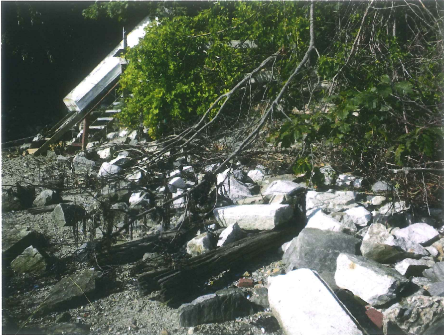
Photograph #4 Miscellaneous granite, concrete & stone along base of slope.
