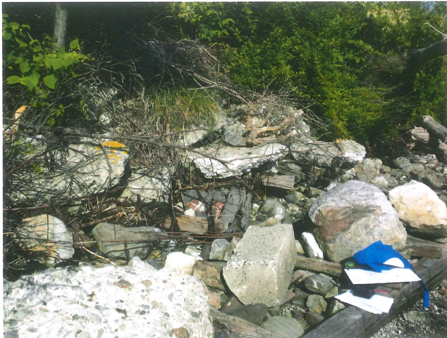
Photograph #6 concrete & stone piled along base of slope.
