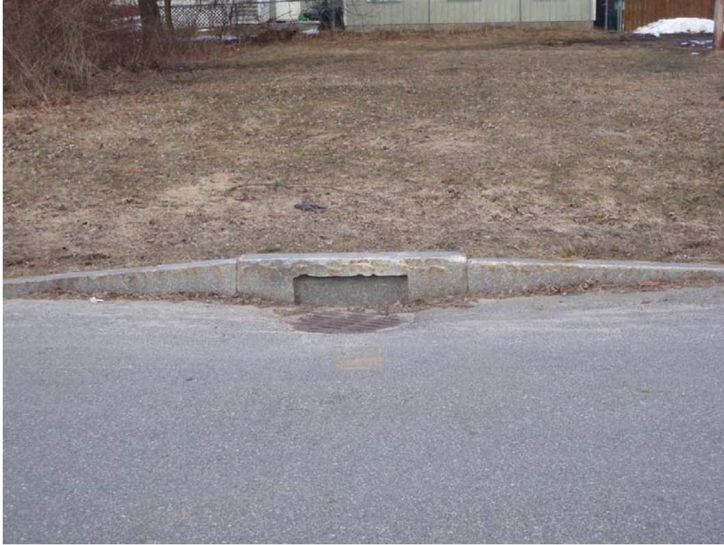
Photo #5 View of existing Catch Basin and Granite Curb Headstone
