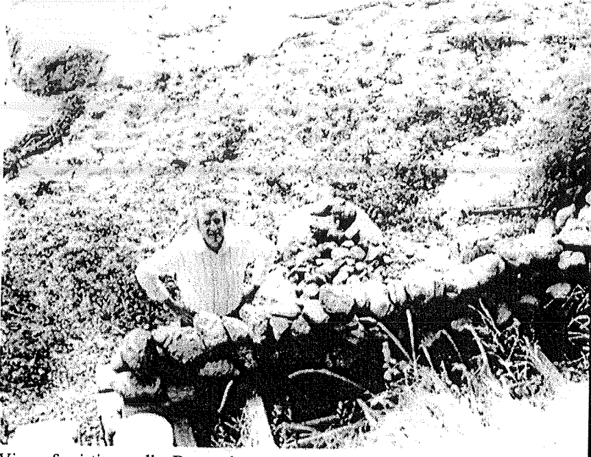
View of existing wall – Date unknown.
