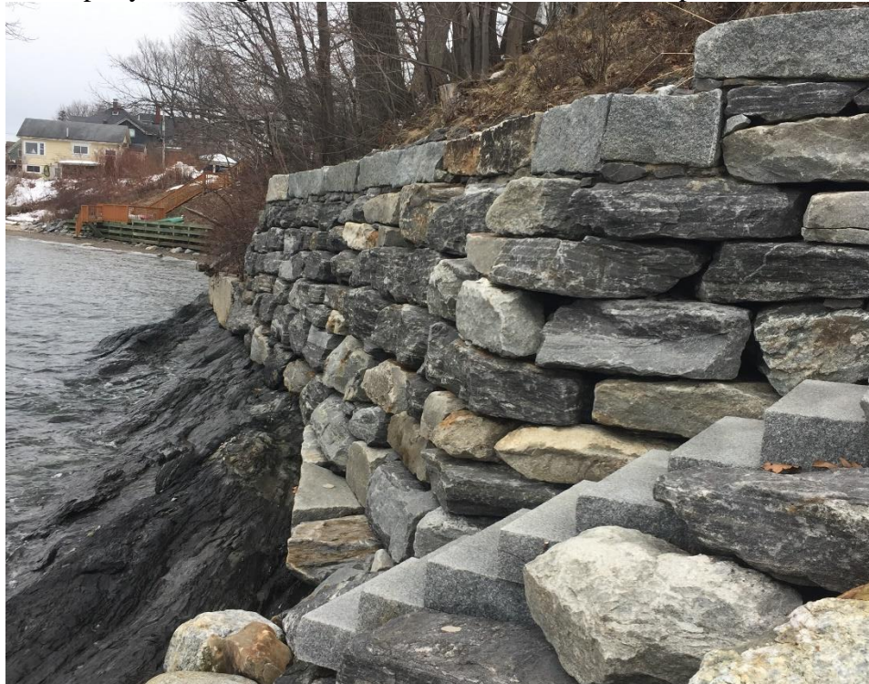
Watson Street Property, neighboring property with pinned granite seawall.
