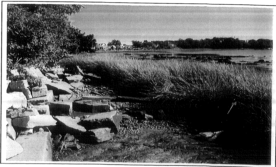
Figure 2. Looking NORTH along toe of the bank. Distance from toe of bank to Spartina alterniflora is 10 feet. Construction of bank stabilization will have minimal impact on intertidal area and will quickly revegetate with native species. [7/27/2010, 8:52 a.m., low tide]
