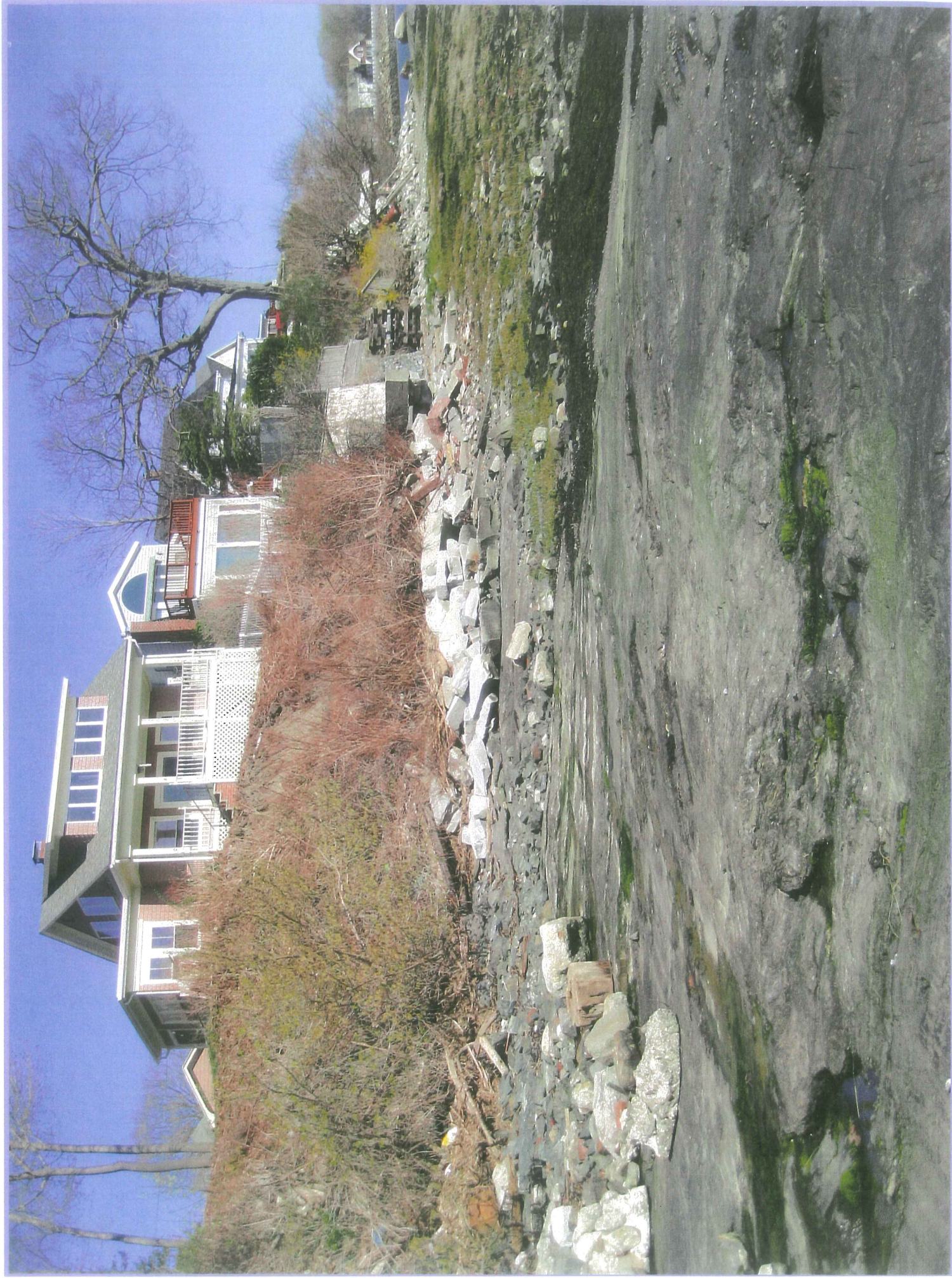
Overview of 6 Island Street, Portland property with failed retaining wall and eroded banking.
