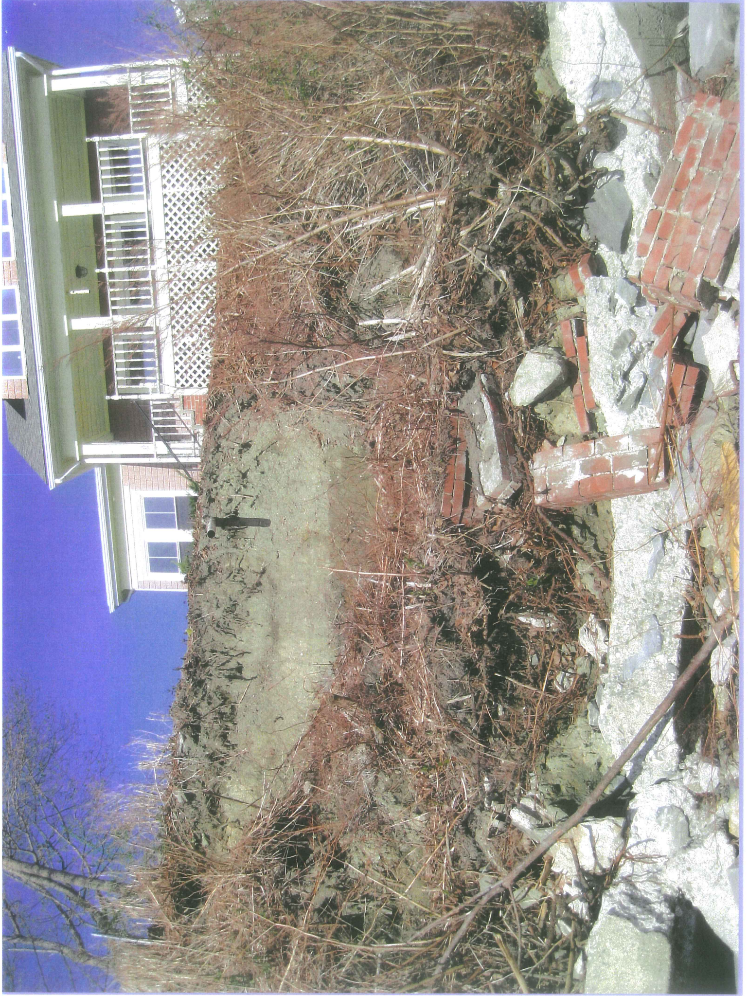
View from shorefront showing failed retaining wall and eroded /slumped bank
