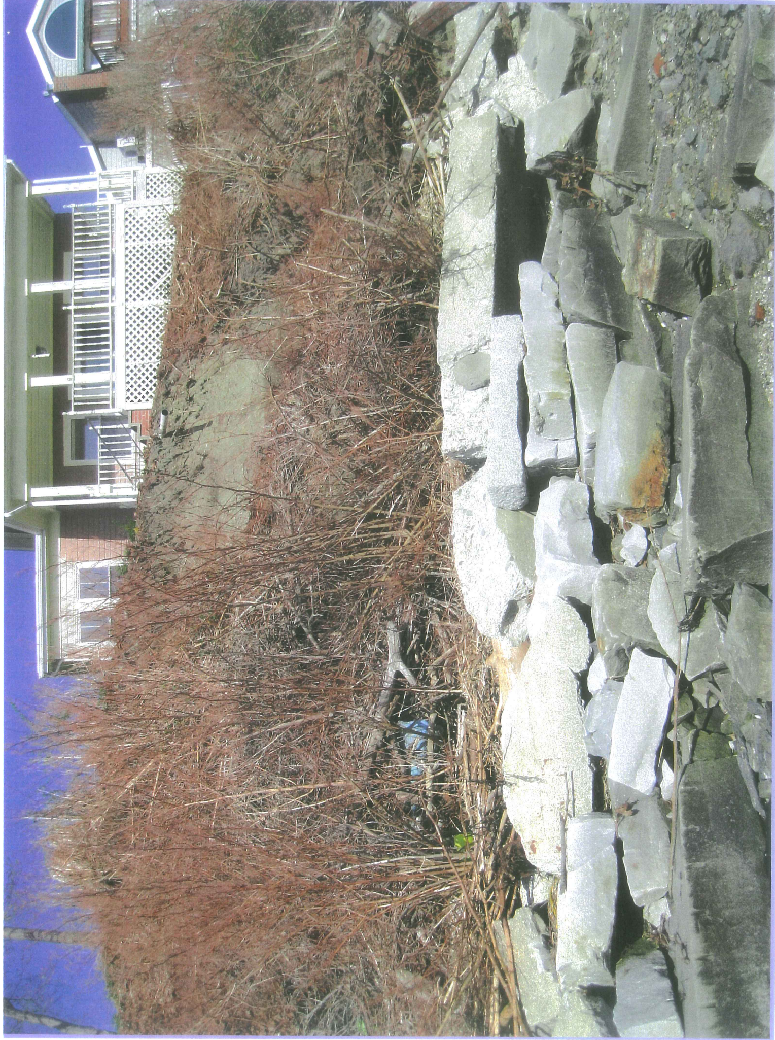
View from shorefront showing eroded banking and failed lower retaining wall
