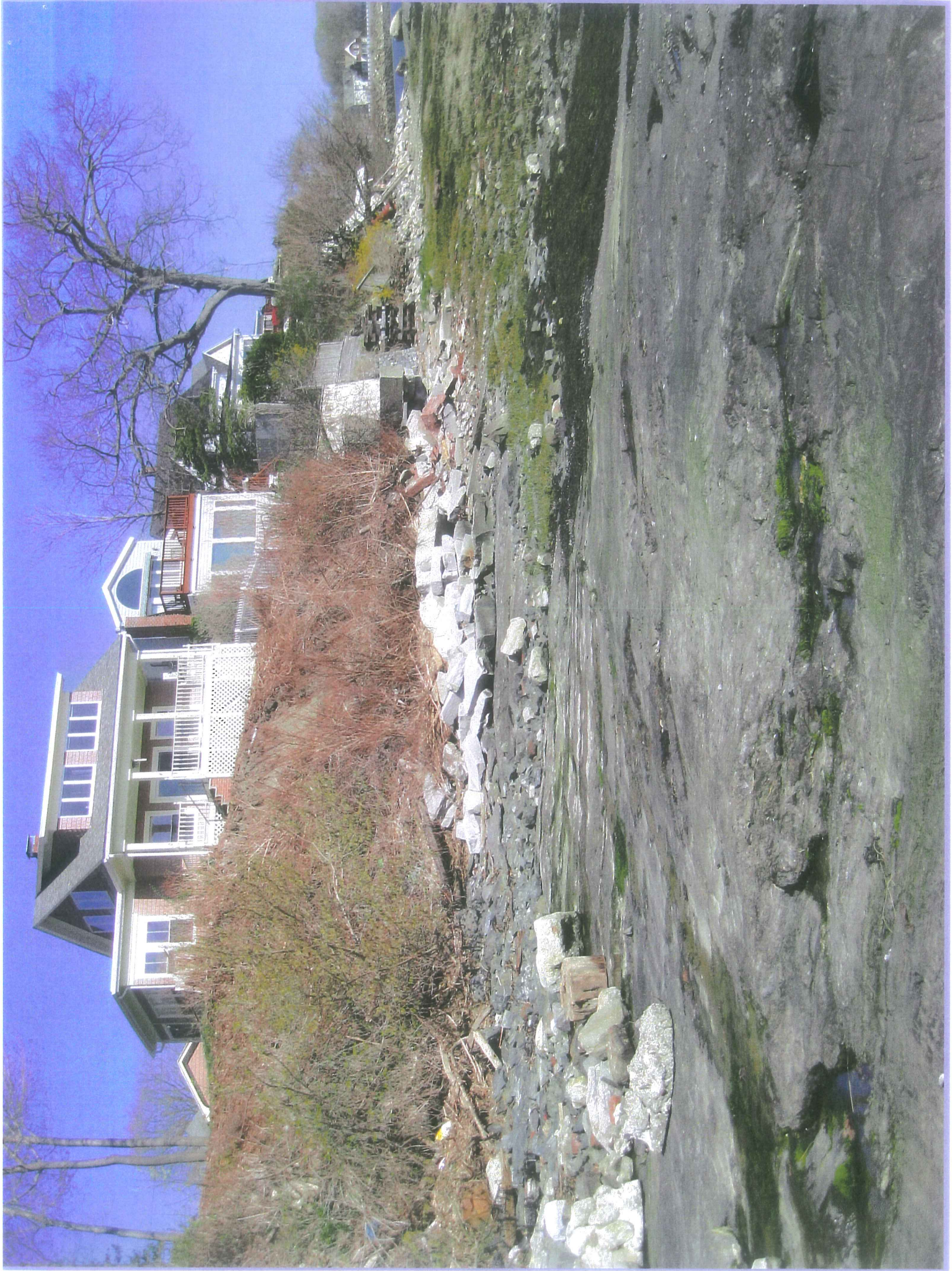
Overview of 6 Teland Street Portland property with failed retaining wall and eroded banking
