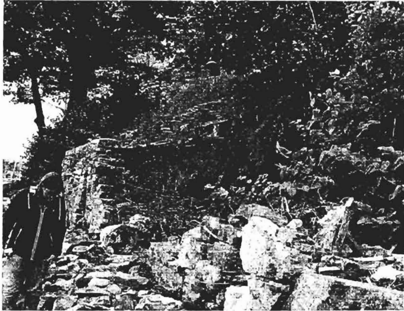
Remaining section of wall showing original slope
