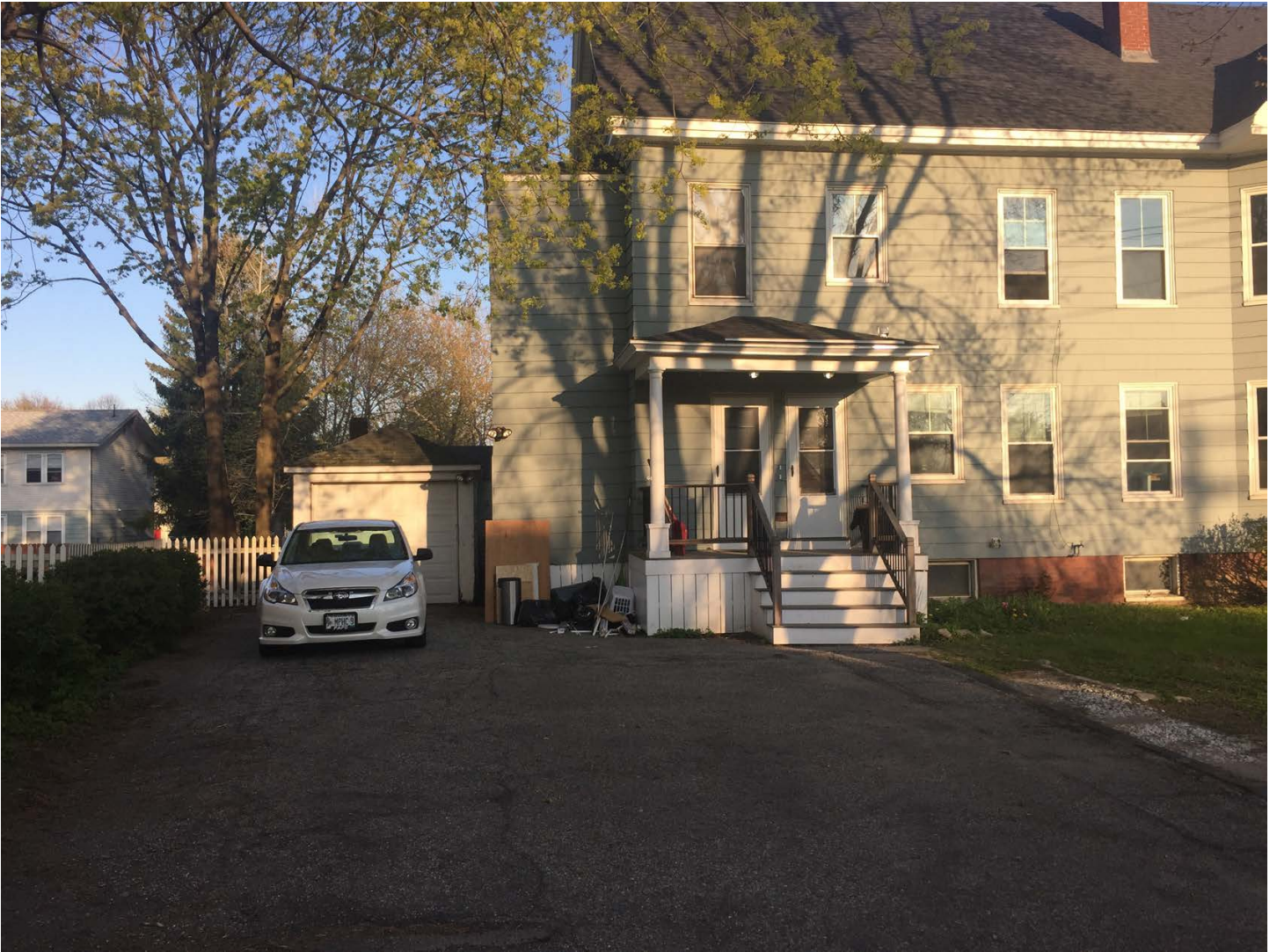
View from end of presumpscot st driveway showing detached garage and primary entrance for existing units.
