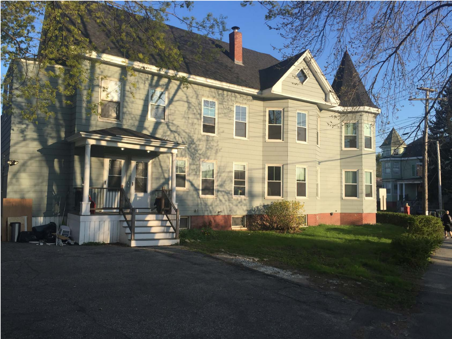
View from end of presumpscot st driveway showing entire presumpscot st facing side of the house
