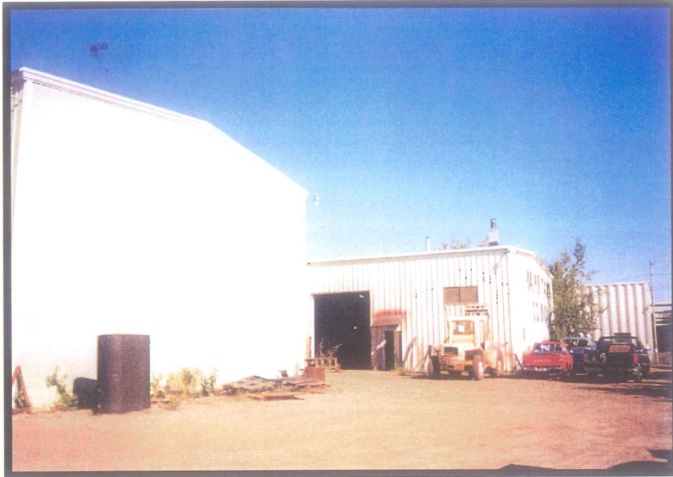
PHOTO 3A: View to northwest, of rear of building; septic tank located where vehicles parked.
