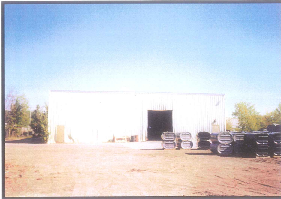
PHOTO 1A: View to north, of 1985b building addition; AST storage area in foreground.
