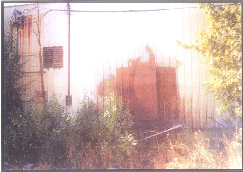
PHOTO 4A: View of painting-booth vent hood on north side of building.
