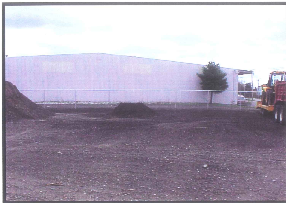
PHOTO 2B: View to south, of Lot 5 portion of site, used for vehicle parking, material stockpiling.
