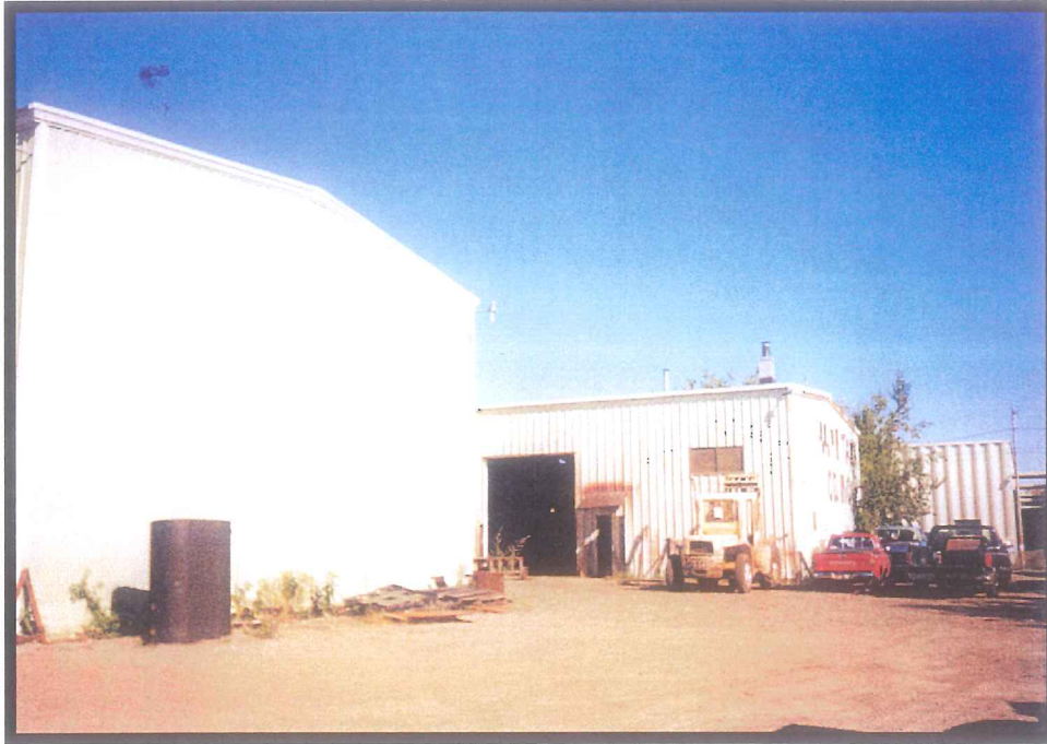
PHOTO 3A: View to northwest, of rear of building; septic tank located where vehicles parked.
