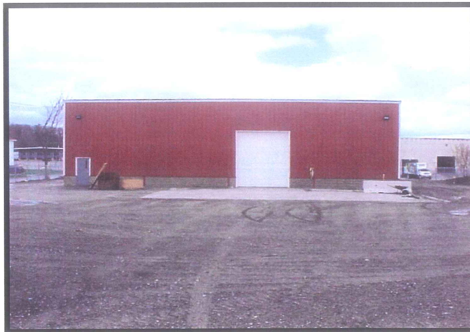
PHOTO 1B: View to north, of current facility upgrade with new siding.
