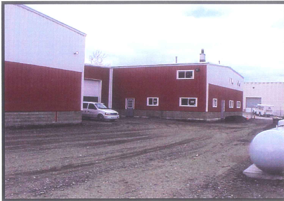
PHOTO 3B: View to northwest, of current rear of building.
