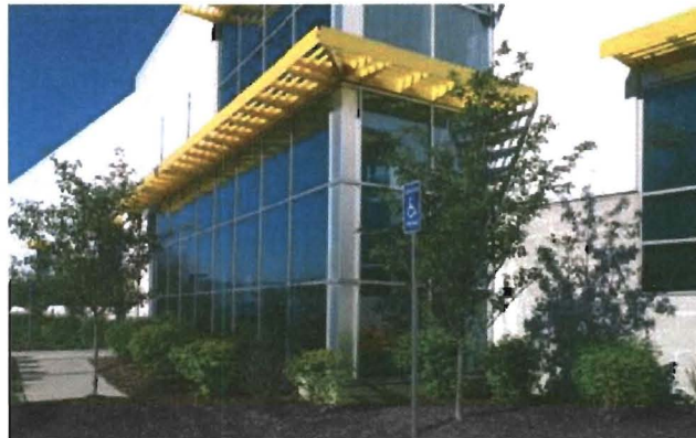
VersaTherm Storefront, 0A Clear Anodized; Owner: Karmann Manufacturing, Plymouth, MI; Architect: DeMattia Group; Tubelite Dealer: Calvin & Company
