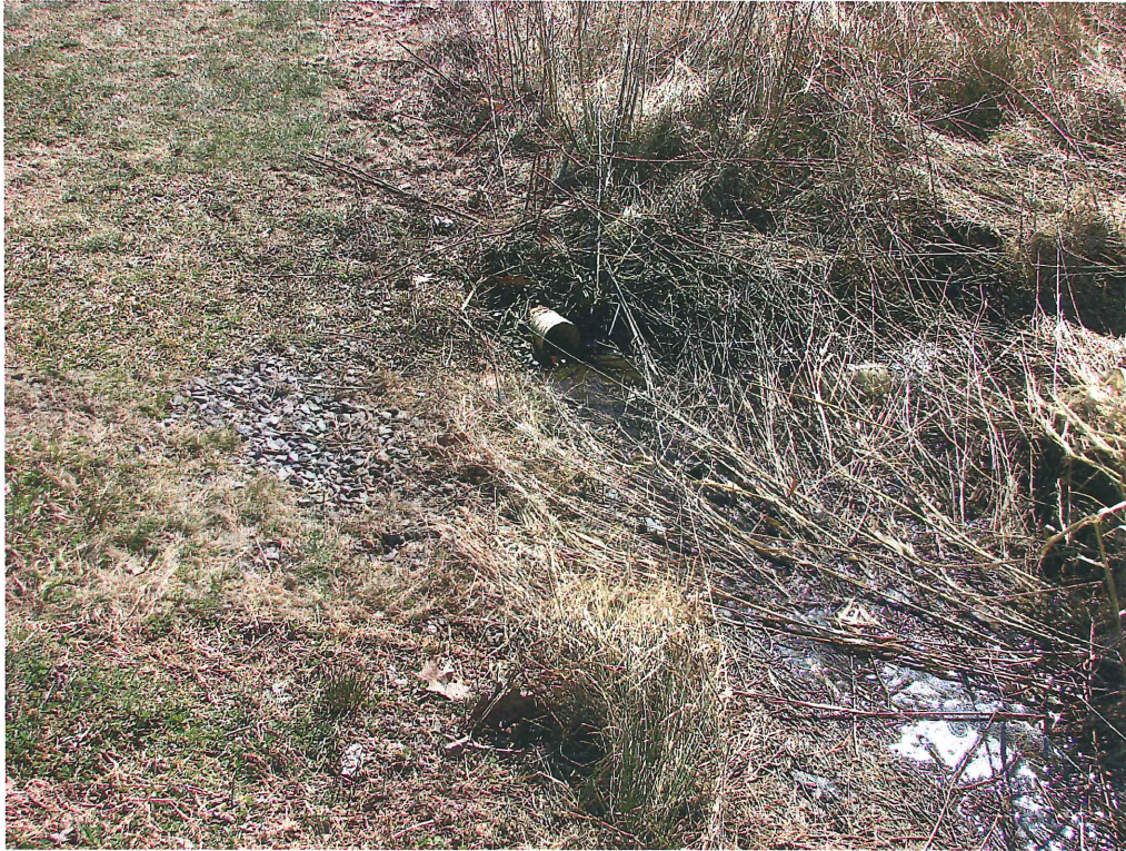
Existing 4" outlet draining southerly side of Eben Hill Drive
