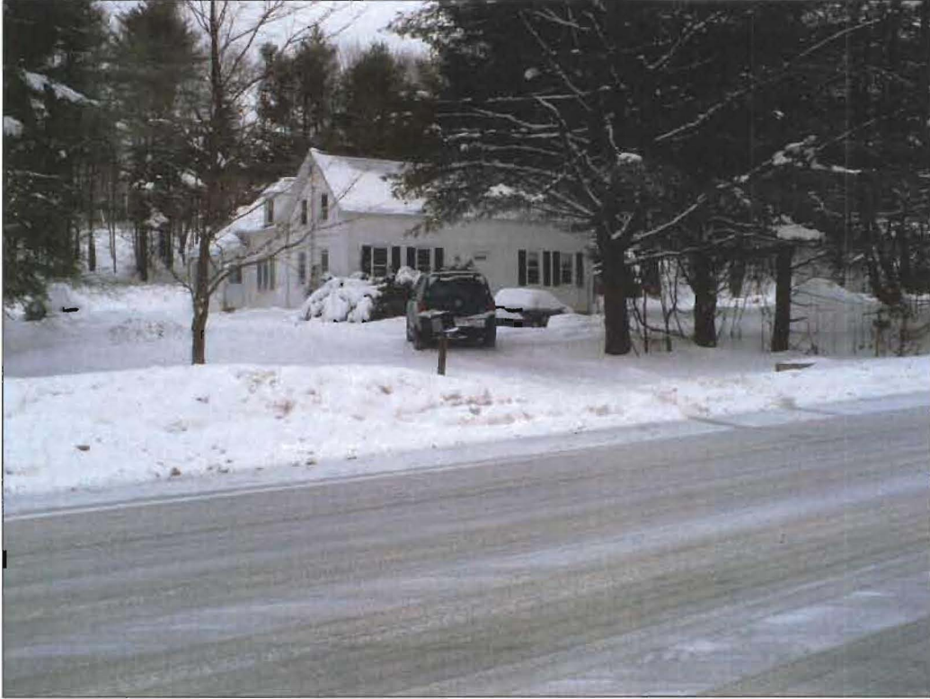
Photo No. 3: 752 Ocean Boulevard.
