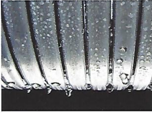
Stainless steel, Viessmann-made Inox-Radial heat exchanger
