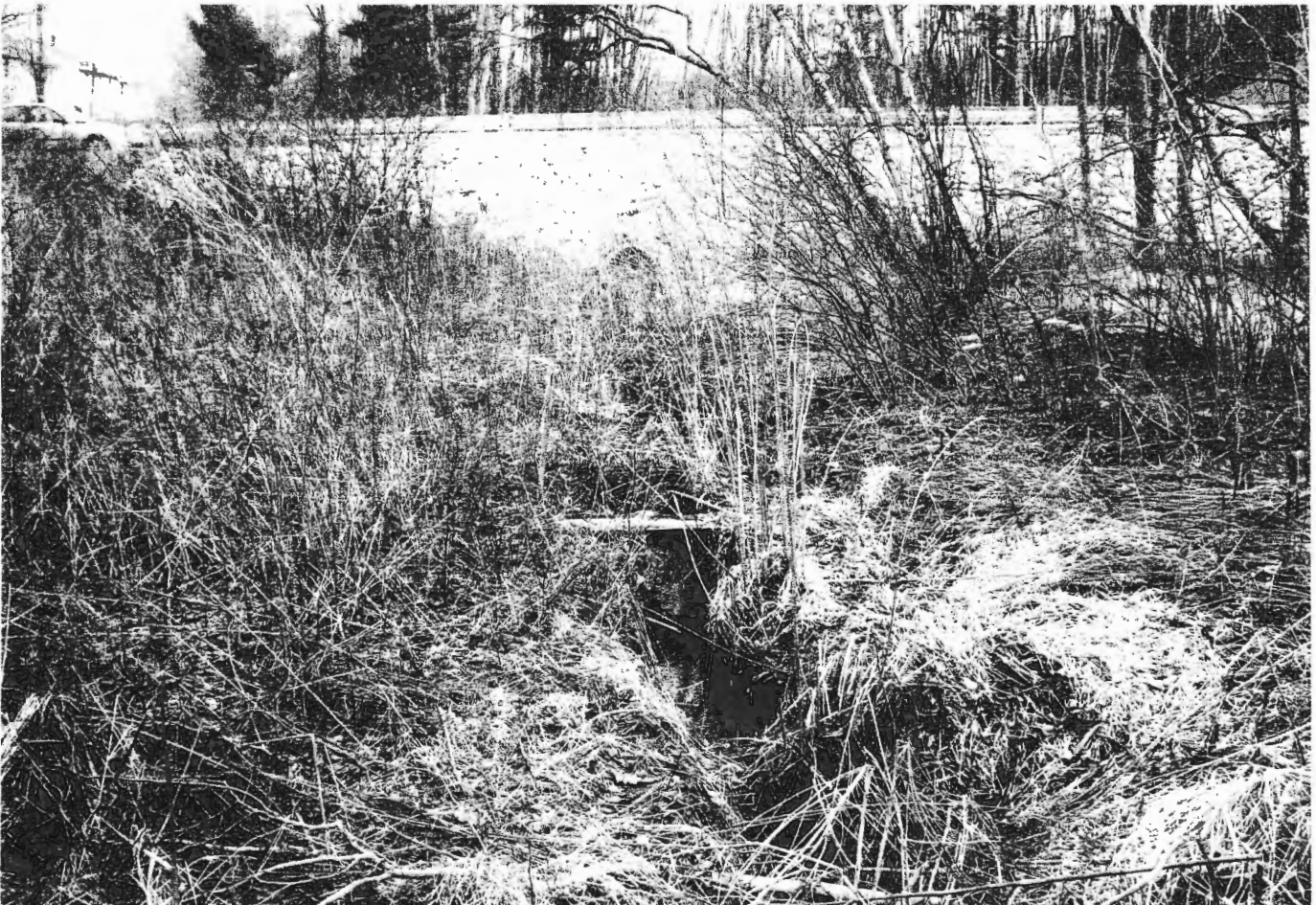
STREAM "LOOKING AT CULVERT"
