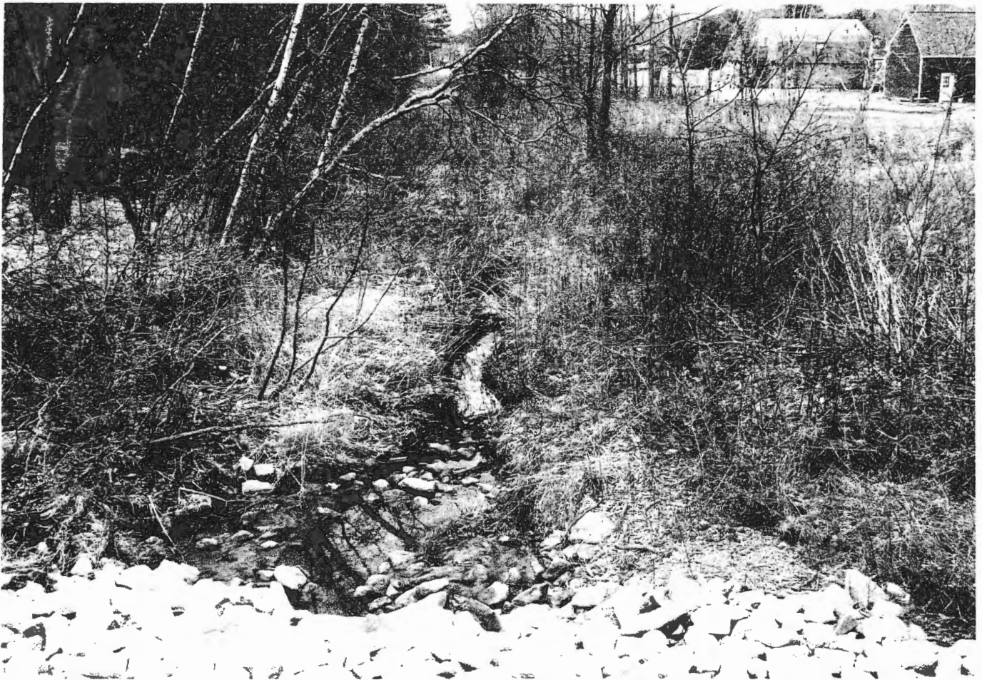
CULVERT FROM DEMEREST STREET
