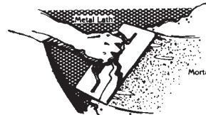
Figure 8 Applying mortar using a plasterer's trowel
