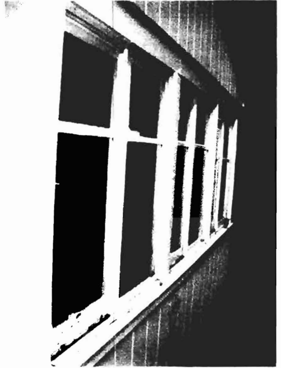
EXTERIOR RIGHT WALL
