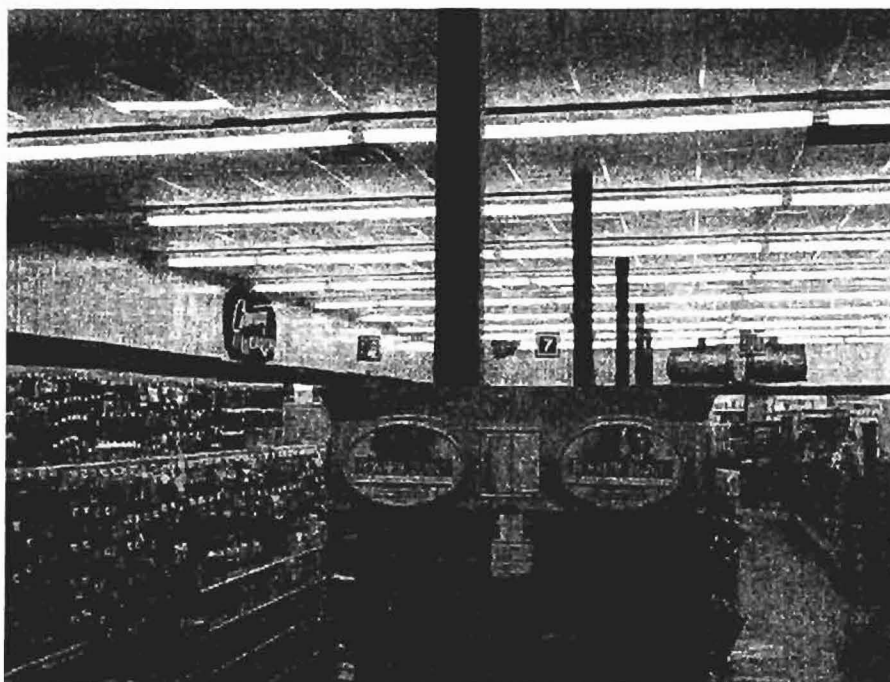
View of retail sales area illustrating ceiling and floor systems.
