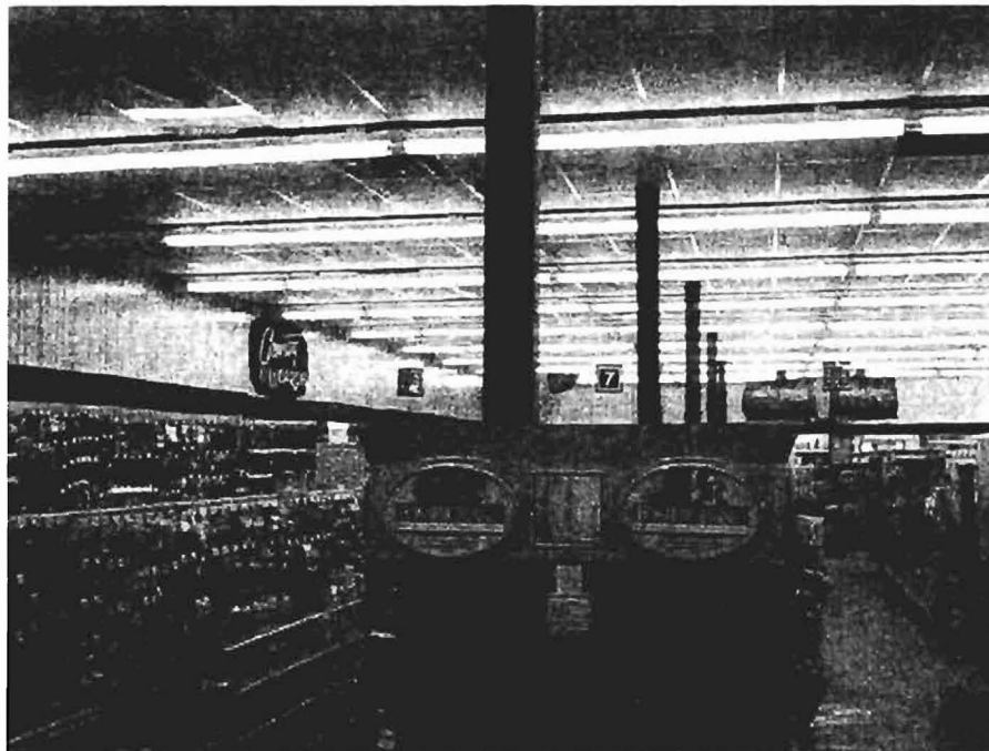
View of retail sales area illustrating ceiling and floor systems.
