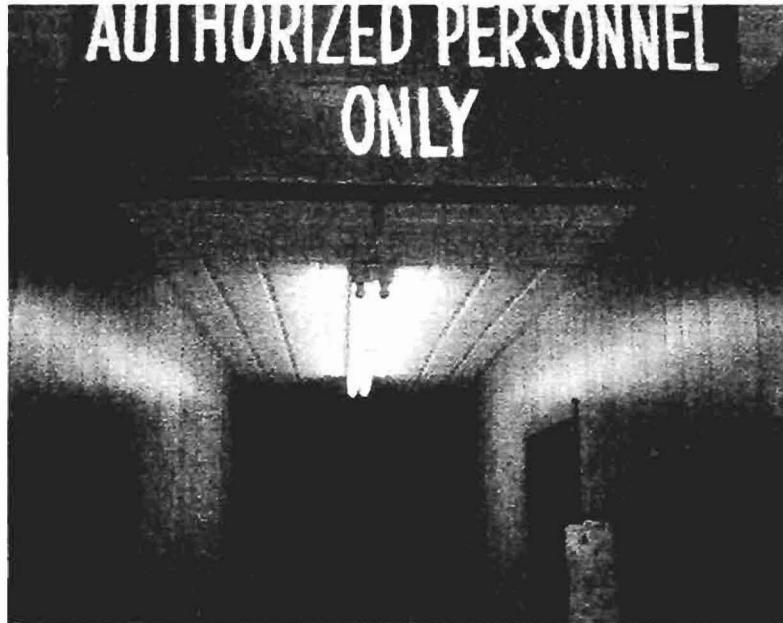
View of hallway area illustrating 2' x 4' ceiling panels.
