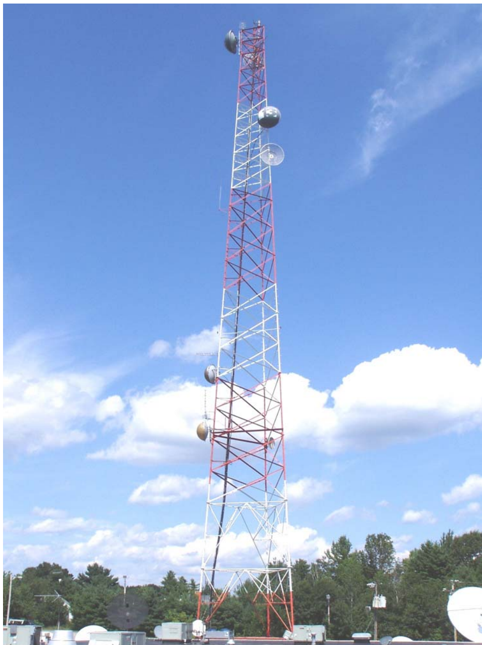
Photo showing overview of 230' Rohn SSVMW self-supporting tower.
