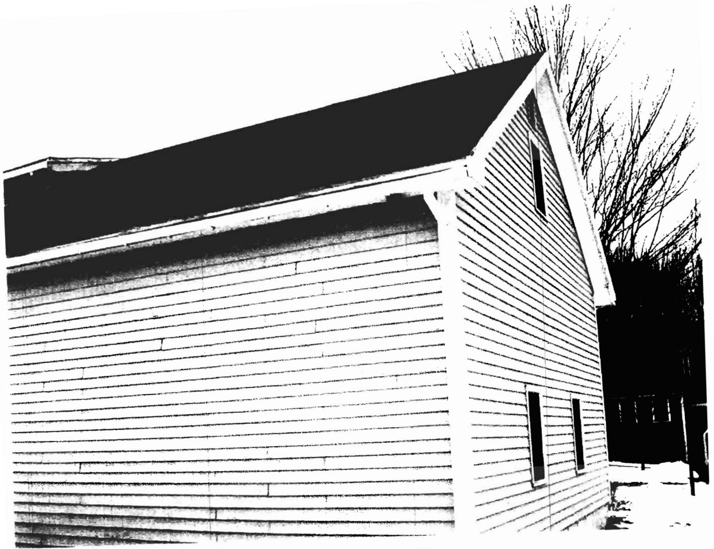
Figure 2 Existing House - Rear
