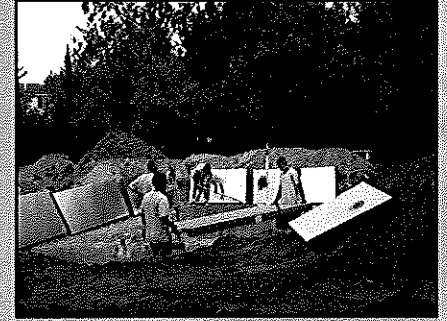
The pool panels are laid out around the excavated hole and ready to assemble.
