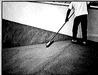
Once the vermiculite has hardened, it is cleaned and prepared for the liner.
