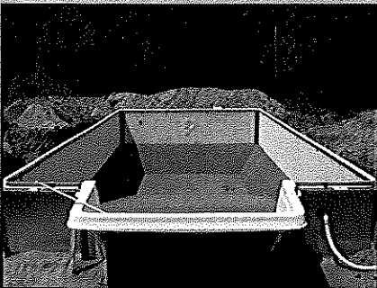
The plumbing is done and base is trowled into place.
