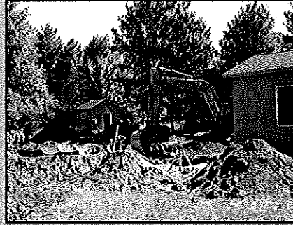
Our excavator will begin digging the pool site to the correct depth and shape.
