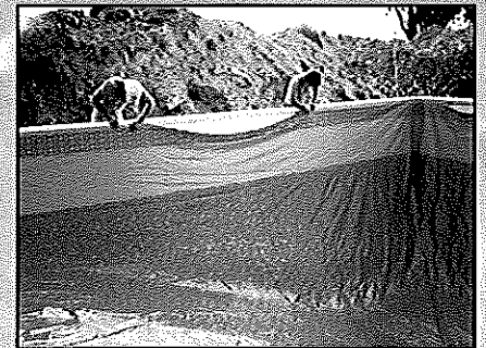
The liner is set in place and the bead is locked into the pool coping.
