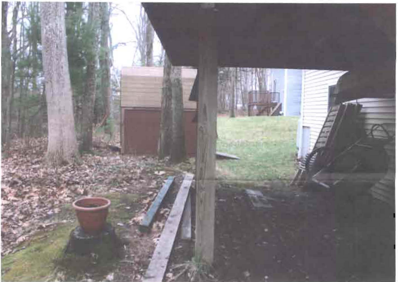
View from northeast under deck
