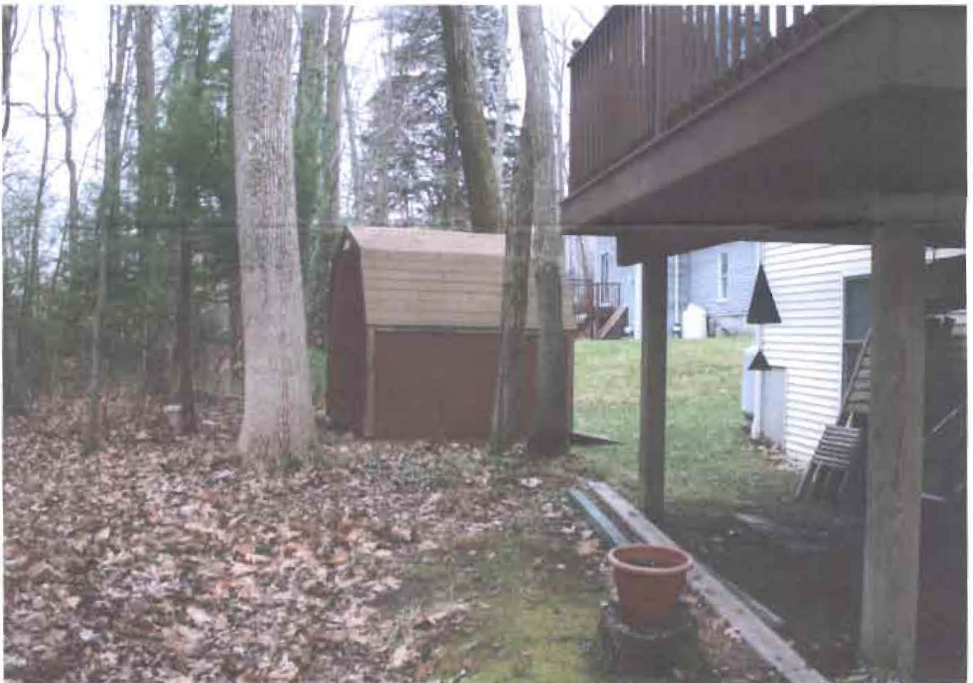
View from northeast behind deck
