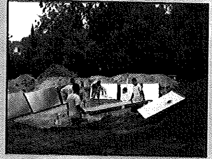
The pool panels are laid out around the excavated hole and ready to assemble.
