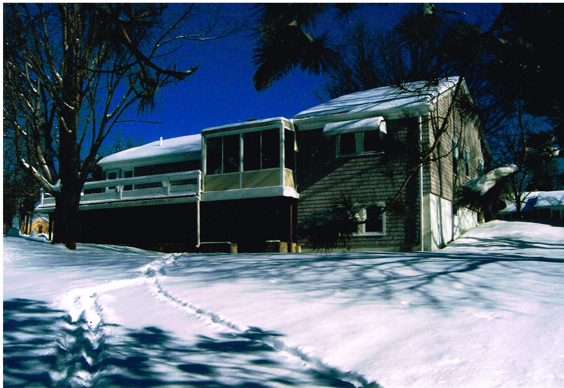
Picture of Existing Sun Room
