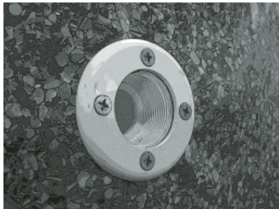
Return faceplate installed.
