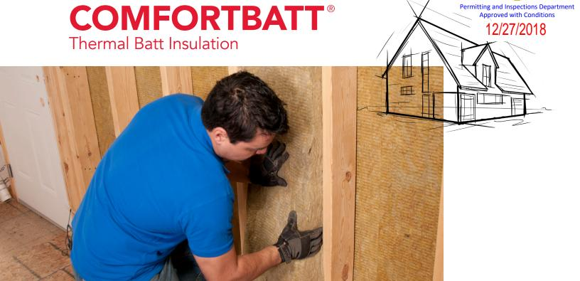
ROCKWOOL COMFORTBATT® is a semi-rigid stone wool batt insulation for exterior wood and steel stud applications in both new construction and renovations.
