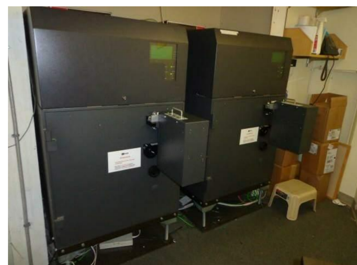
RELOCATE ONE ATM. RELOCATE AND LOWER SECOND ATM TO COMPLY WITH 2010 ADAAG.
