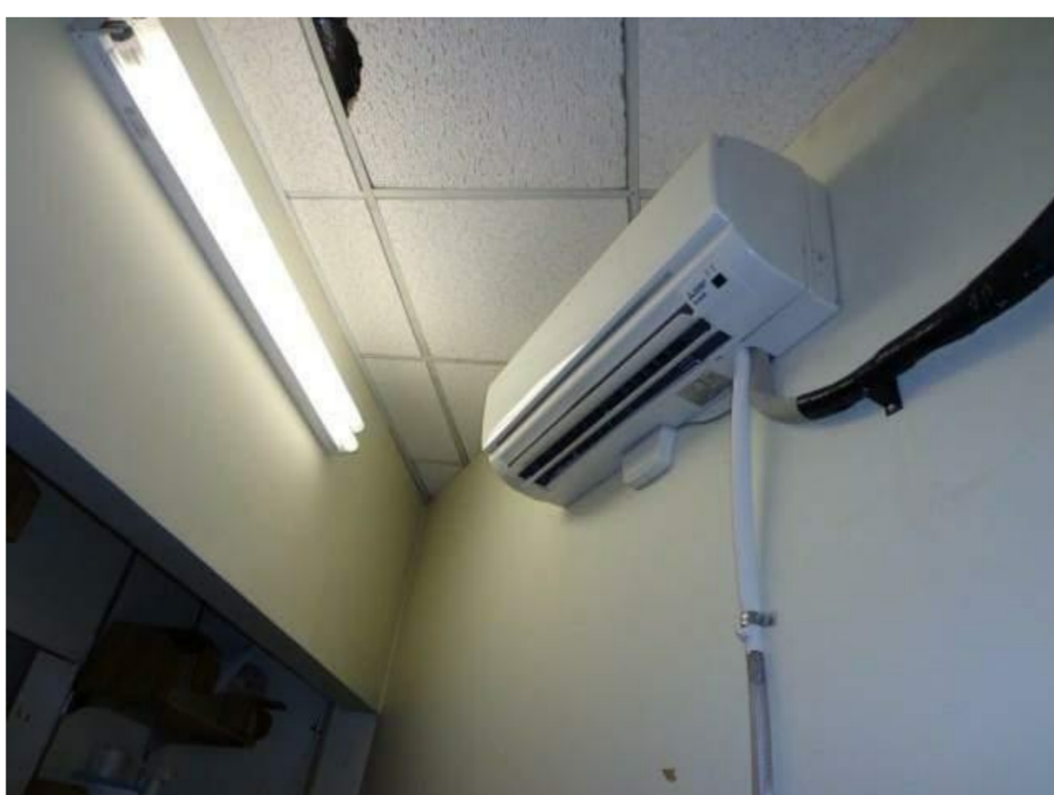
ATM ROOM - RELOCATE EXISTING HVAC UNIT .
