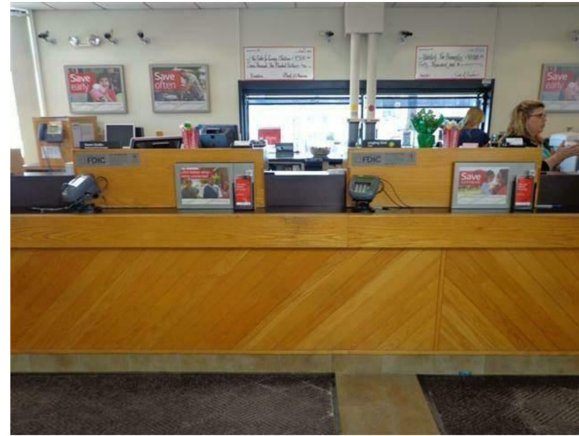
TELLER STATION TO BE MADE ADA COMPLIANT
