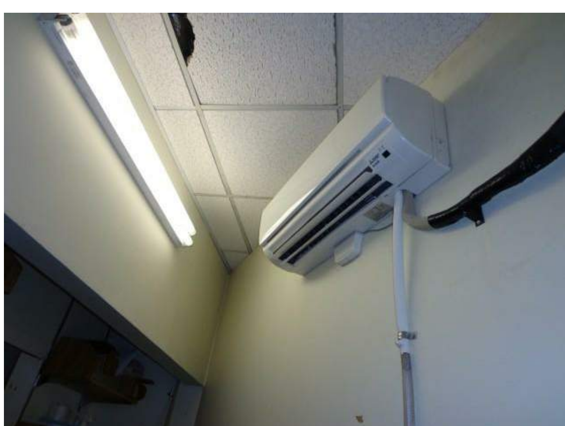
ATM ROOM - RELOCATE EXISTING HVAC UNIT.
