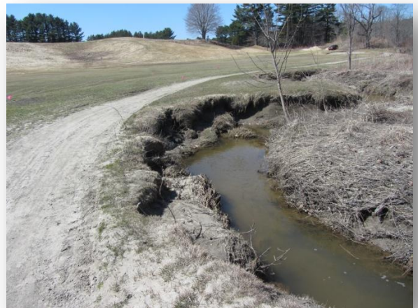
Zone 3 – Looking north from footbridge.
