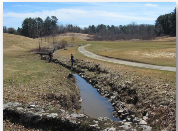
Zone 4 - Looking south from the stone bridge.
