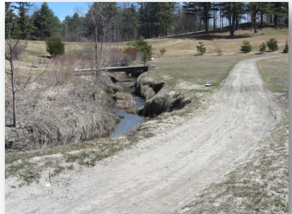
Zone 2 – Looking south east.
