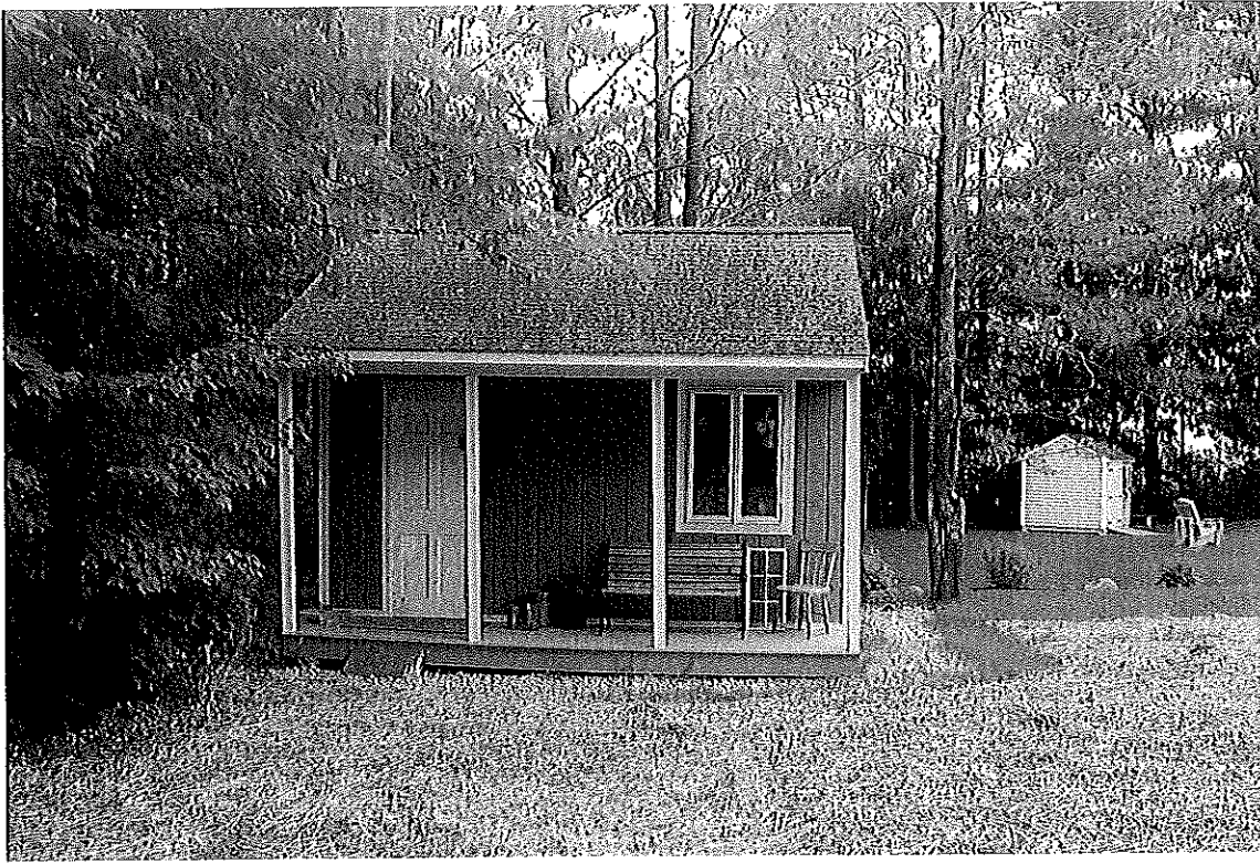
Front view of shed
