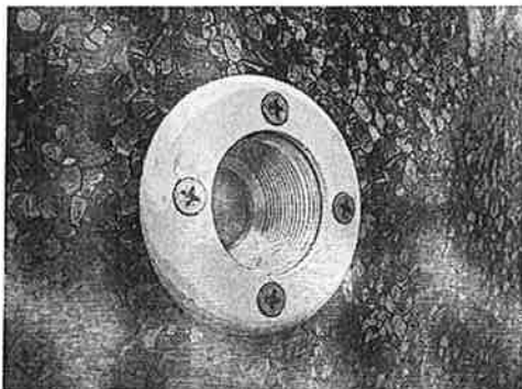
Return faceplate installed.
