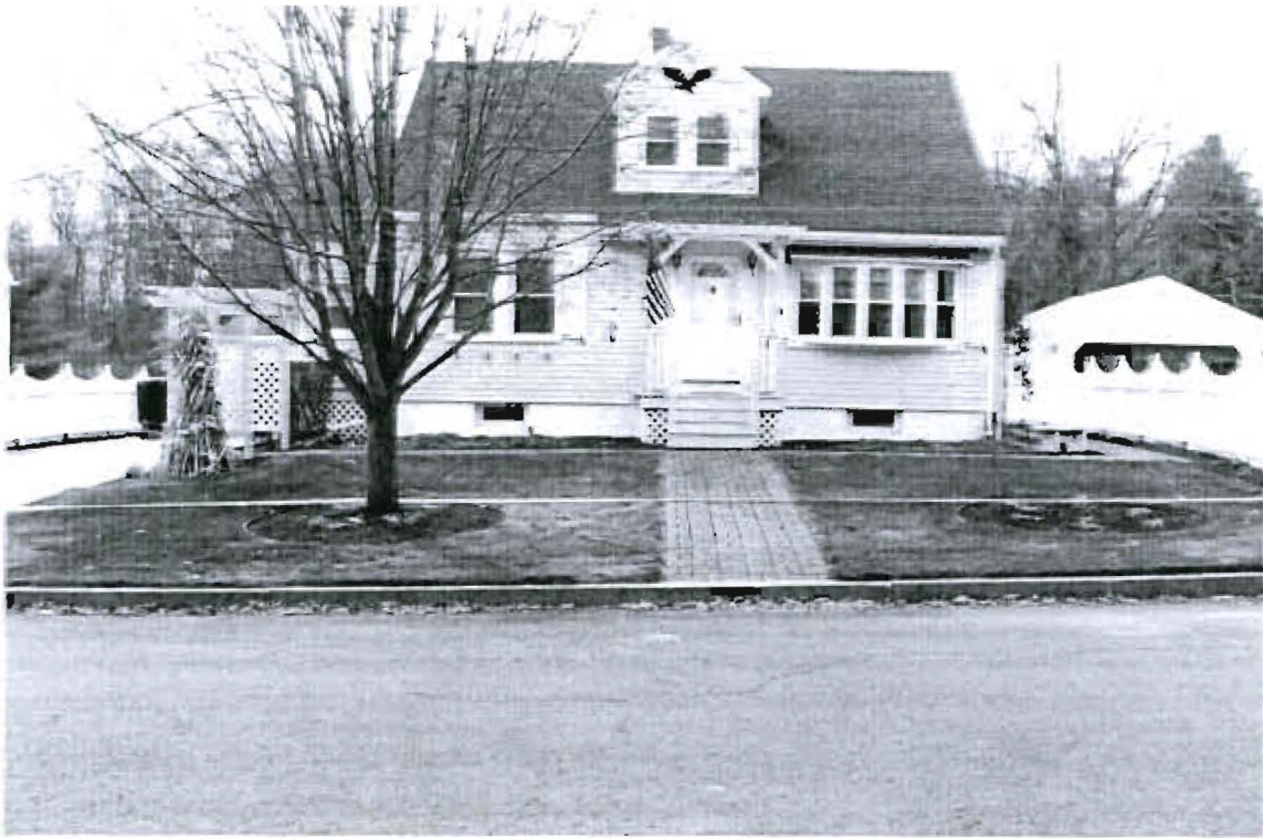
Picture 1 Full view of house with existing porch.
