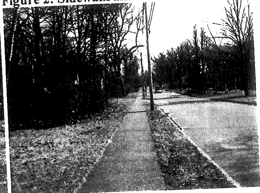
Figure 2: Sidewalk and Overhead Utilities
