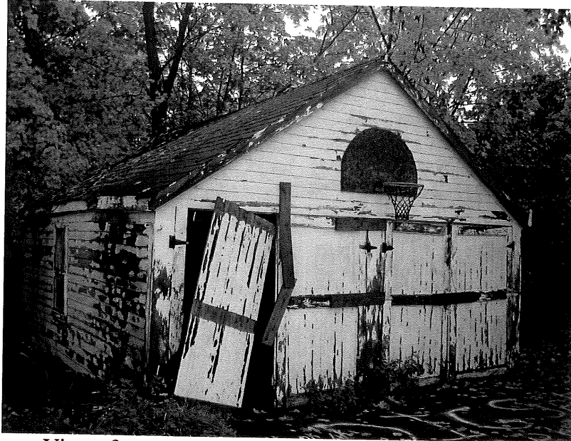
View of garage structure assessed during this activity.
